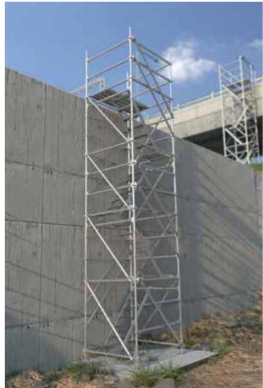
Stair tower site access
